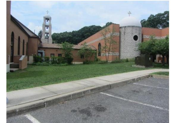
Stormwater currently pools in several locations in the parking lot. Downspouts can be disconnected into a rain garden, and pervious pavement can infiltrate runoff from the parking lot. A preliminary soil assessment suggests that the soils have suitable drainage characteristics for green infrastructure.
