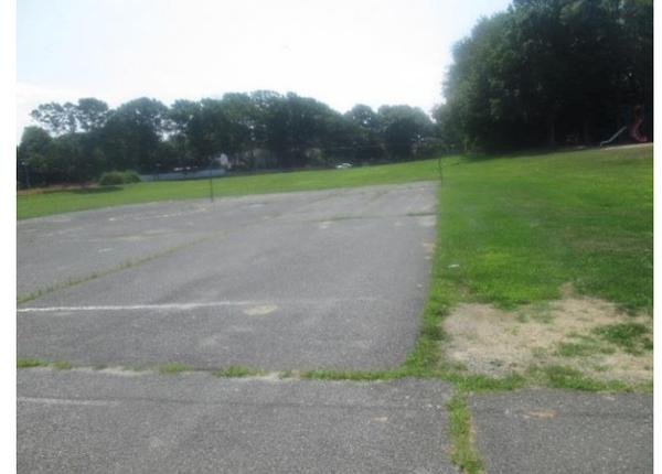
Parking spaces can be replaced with porous asphalt to infiltrate runoff. A rain garden can be installed adjacent to the building to capture, treat, and infiltrate roof runoff. A preliminary soil assessment suggests that the soils have suitable drainage characteristics for green infrastructure.
